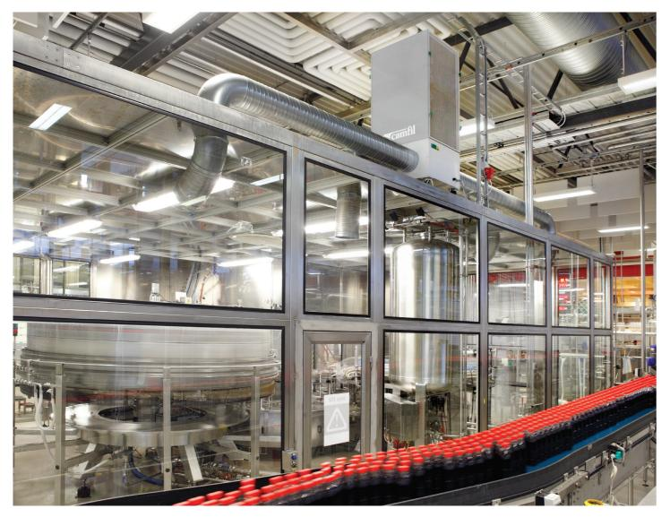
The picture shows a bottling plant that requires a lot of clean air behind its glazed surfaces. Air from outside is drawn into the air purifier and passes through the high-efficiency HEPA filter before it is directed into the bottling plant.
