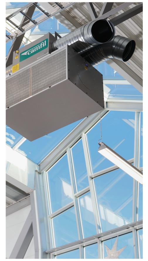
A ceiling-mounted air purifier efficiently purifies the air of nanoparticles as well as of large visible bits of dust. At the same time, the air is remixed, which provides a higher average temperature at floor level.
